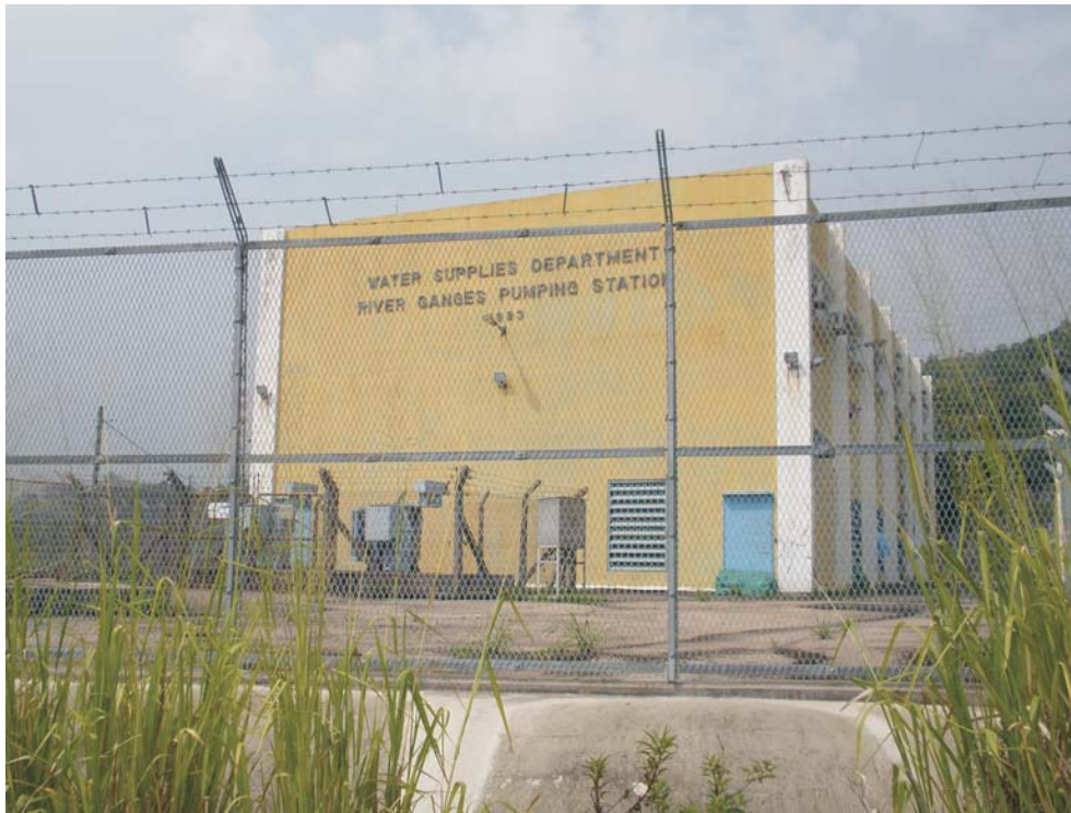
River Ganges water pumping station
