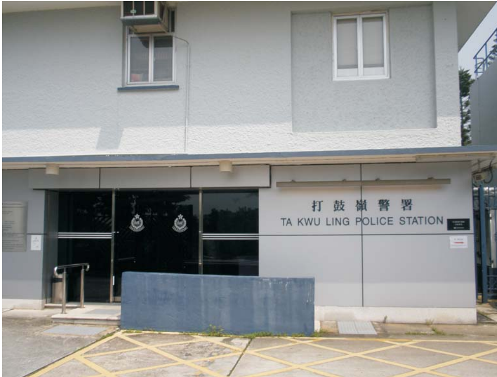
Ta Kwu Ling Police Station
