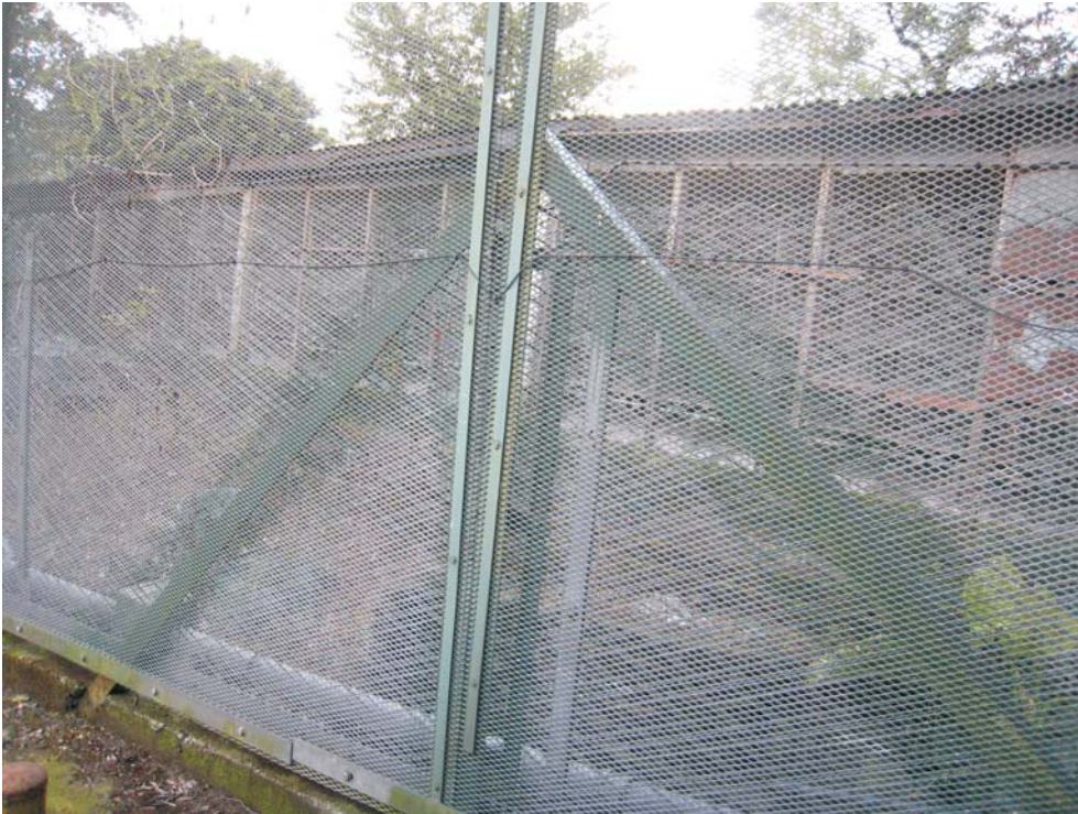
Abandoned poultry farm in Site 1
