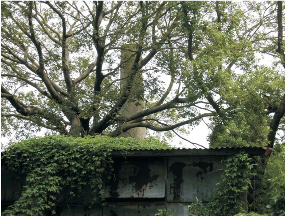
An industrial site with an air emission stack in Site 4
